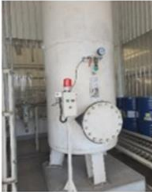
Gambar 20. Panel Sistem Monitoring Ala
